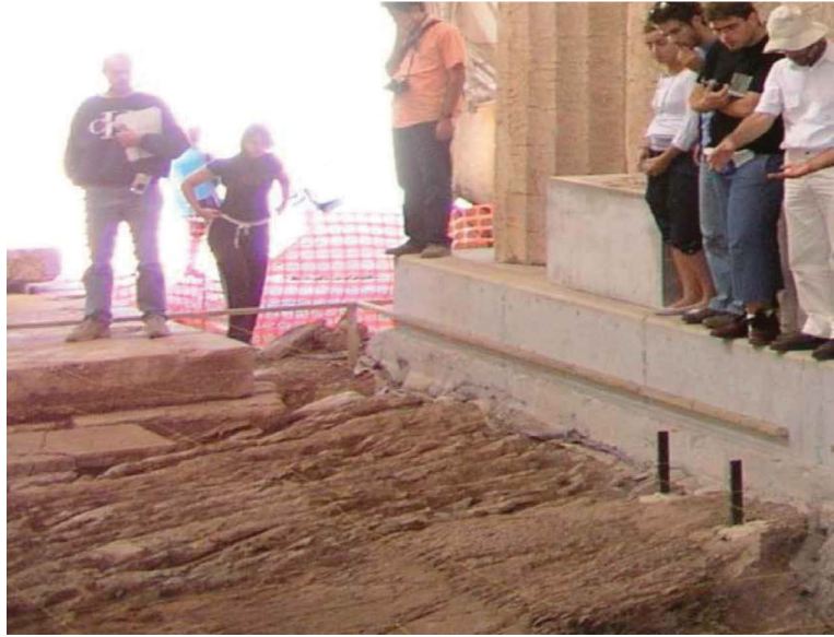
Fig. 17: View from the southeast of the bedrock underlying the central part of the north façade of the Bassai monument. The linear edge of the cavity cut in the rock is visible at the bottom of the photograph.
