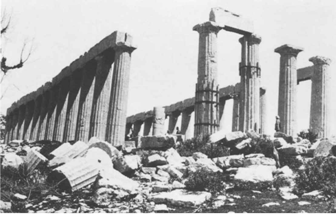
Fig. 53: The temple from the southwest, c. 1891. The hoops around the two columns on the south side are visible.
